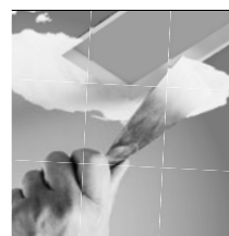
skimmed into plasterboard ceiling (trimless)
