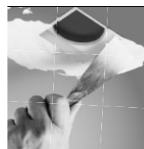
skimmed into plasterboard ceiling (trimless)
