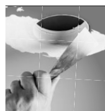
skimmed into plasterboard ceiling (trimless)
