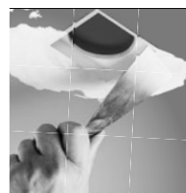
skimmed into plasterboard ceiling (trimless)
