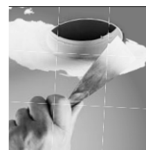
skimmed into plasterboard ceiling (trimless)
