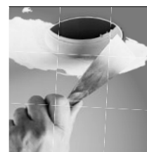
skimmed into plasterboard ceiling (trimless)
