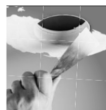
skimmed into plasterboard ceiling (trimless)
