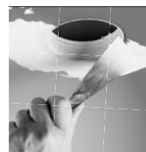
skimmed into plasterboard ceiling (trimless)
