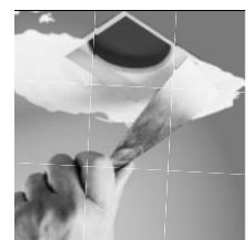
skimmed into plasterboard ceiling (trimless)
