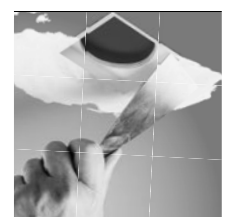
skimmed into plasterboard ceiling (trimless)
