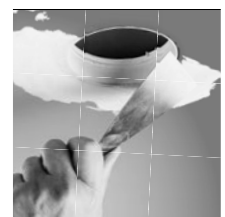
skimmed into plaster-board ceiling (trimless)
